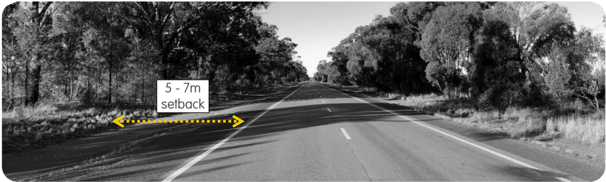
Figure 9 Newell Highway Facing North-East Adjacent the Subject Site
