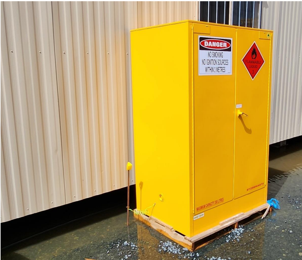
Photograph C.7 Chemical storage within locked cabinet
