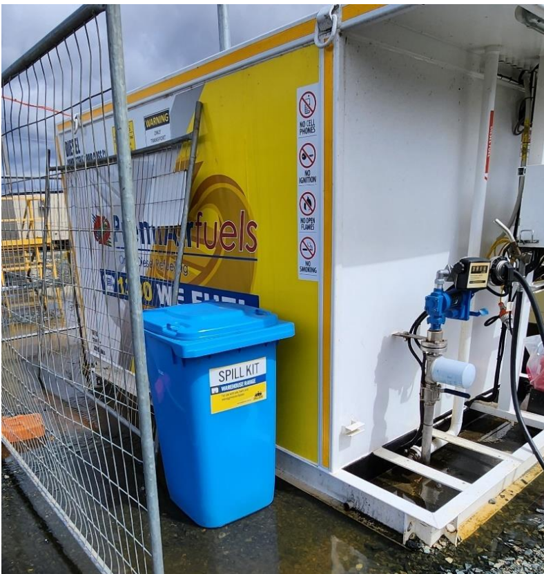
Photograph C.6 Fuel storage fenced bunded and spill kit located nearby
