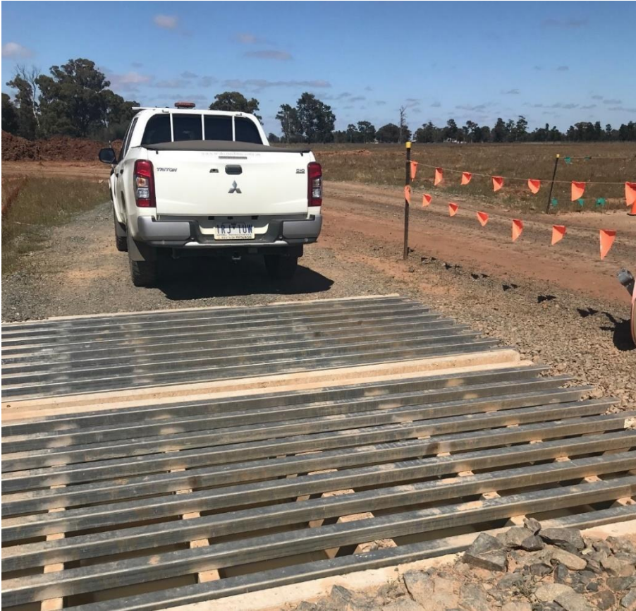
Photograph C.13 Rumble grid cleaned out and re-instated
