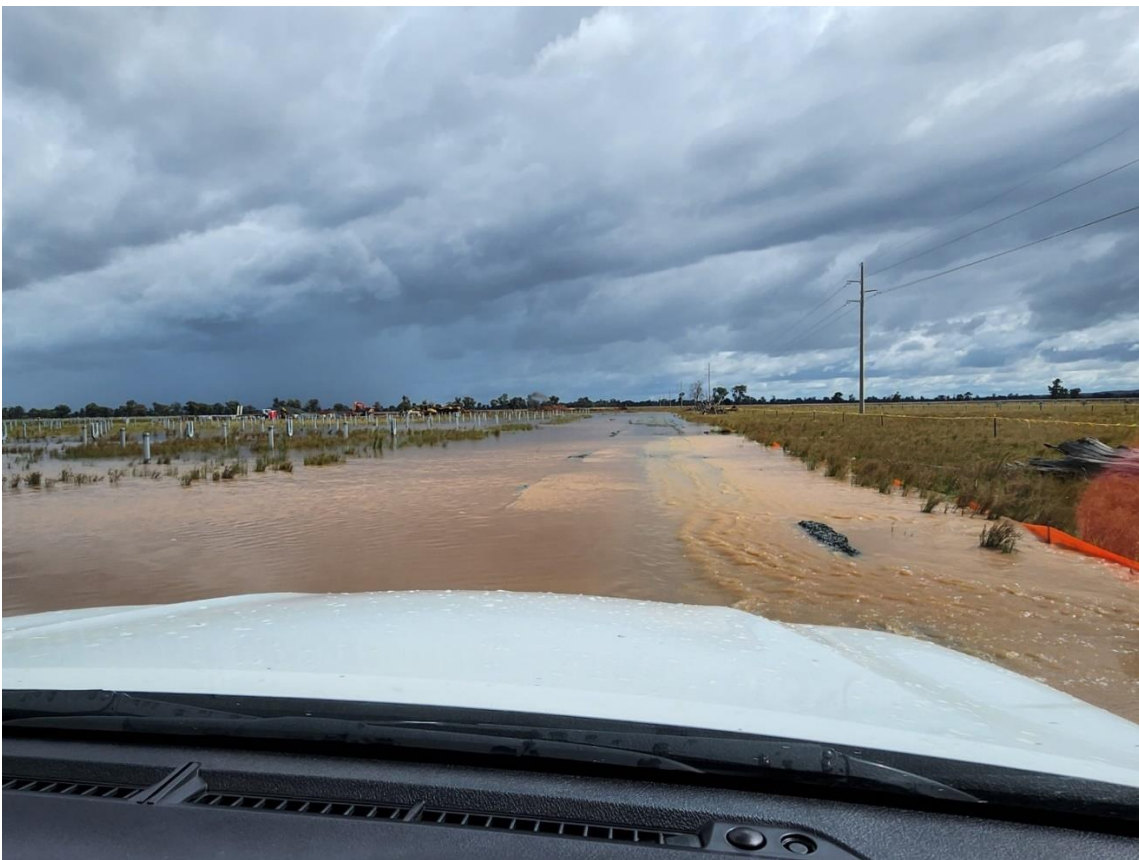
Photograph C.10 Internal roads are gravel, existing sediment fence during extreme weather event
