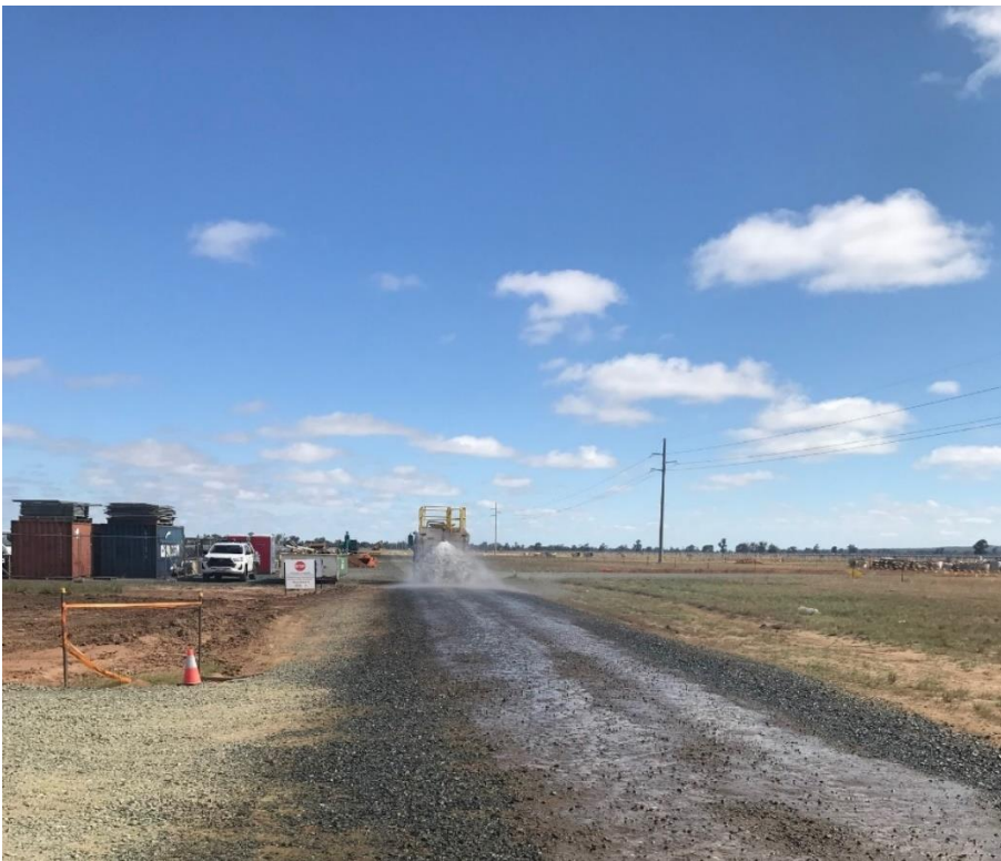
Photograph C.14 Water truck in use for dust prevention
